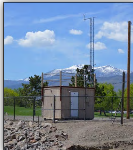
Figure 8 South Reno Monitoring Site
