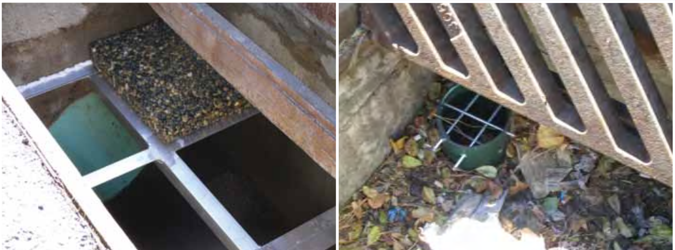
Figure 1: A Type 4R catch basin, showing the insert frame with a single paver on the frame above the outlet pipe (left) and the Xeripave insert with the 5 pavers and overflow unit (right).
